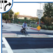
MEDIAN ISLAND TRAFFIC DIVERTER
